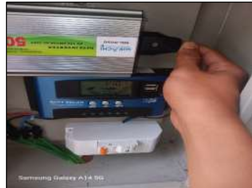
Gambar 4 10 Wiring Inverter 500W Ke MCB
