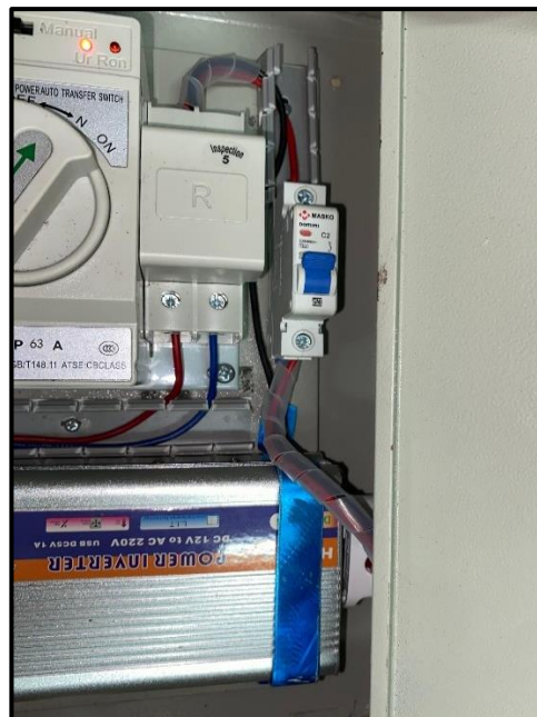
Gambar 4. 4 Wiring Inverter 100Watt ke ATS 220VAC
